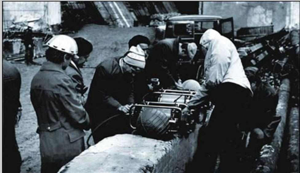
The construction of the Sayano-Shushenskaya hydro-electric power station. Members of the Chair of Television are assembling an experimental submarine television installation in one of the workshops. (1982).
