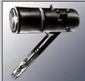
One of the first models of the super-conoscope-the transmitting television tube, made in P.Shmakov's laboratory. 1937
